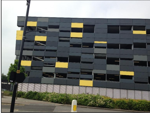
Figure 11 Multi-storey car park
