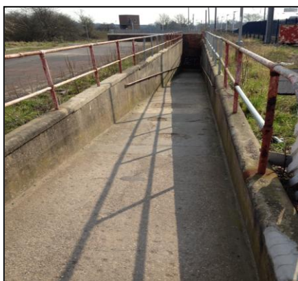
Figure 7 – Ramp for subway to the south side of Retford Rail Station
