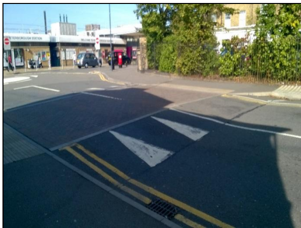
Figure 2 Raised table crossing point, Station Road (near Great Northern Hotel Building)
