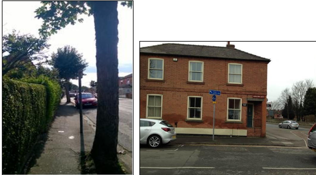
Figure 9 Cracked pavement and limited signage on Appleton Gate
