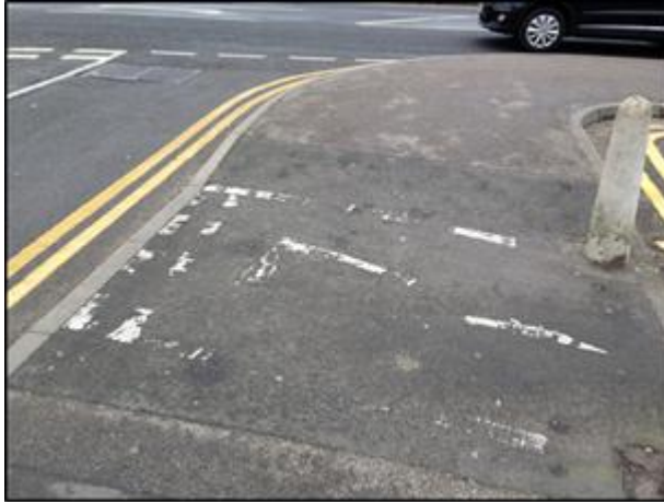
Figure 13 Uneven and faded cycling markings at Lincoln Road
