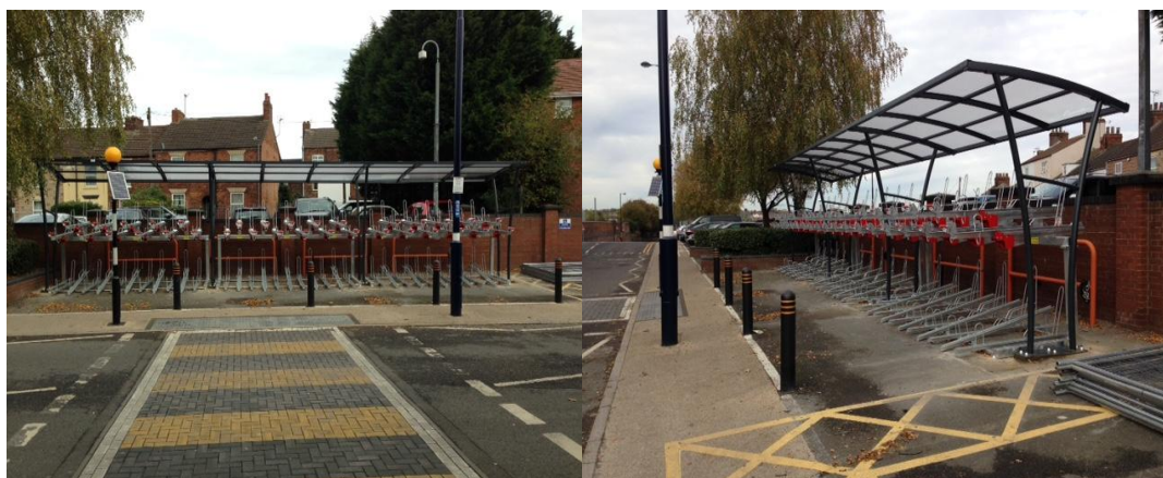
Double Tier Cycle Parking which is now located opposite the main entrance.
