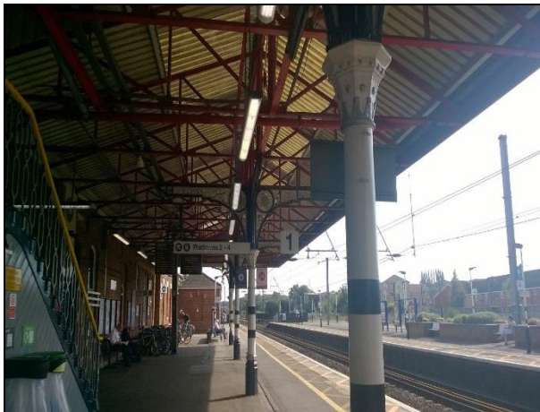
Figure 3 Platform 1 Concourse / Step Bridge
