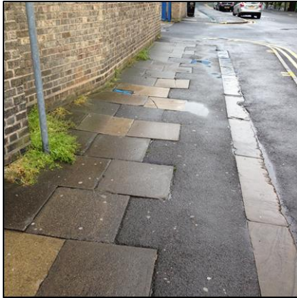
Figure 7 Uneven and pitted pavements
